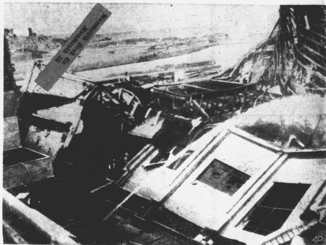
Here's a view of the twisted wreckage of an unfinished $1,250,000 hangar at LaGuardia Field, New York, after flames swept through it, causing part of the roof to collapse. Damage estimates ranged from $250,000 to $1,000,000.
