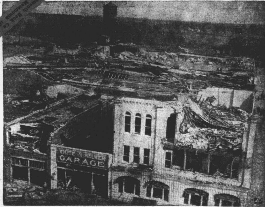
A savage tornado roaring into Albany, Ga., "like a thousand freight trains" left such scenes of devastation in its wake as this. This after-tornado view shows how the mighty brick stores and caused tops of business houses to cave in. (More tornado pictures on page four).
