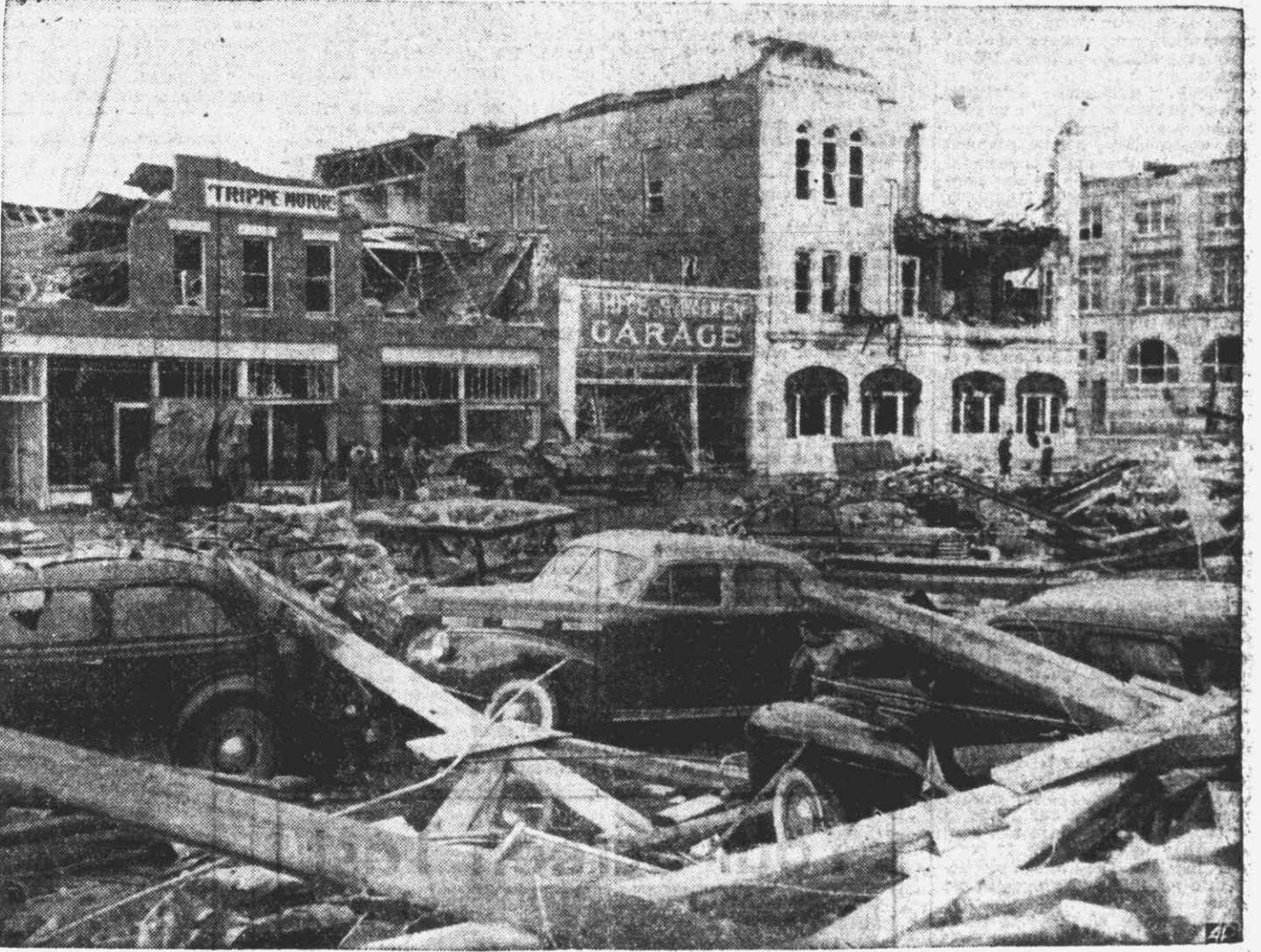
Falling buildings bowled over and shattered by a terrific tornado at Albany, Ga., created such havoc scenes as this. The blow was tough on automobiles as seen here. Crumpling buildings crushed automobiles in the street. This shot of a principal street in Albany shows demolished cars and skeletons of buildings on all sides.
