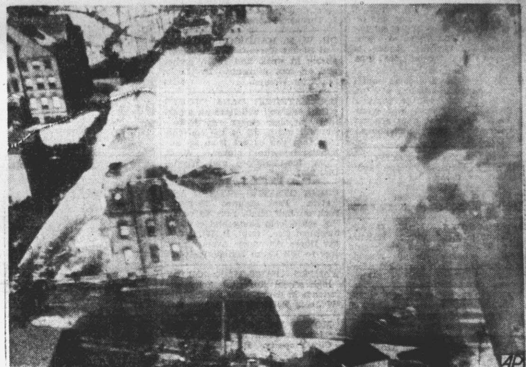
Five hundred and forty pupils and 20 teachers escaped without injury as flames raged through the Point Street grammar school in Providence, R. I. One fireman was injured by a falling wall. This air view, taken at the height of the fire, shows firemen battling to bring the flames under control. Many of the children in third-floor rooms were forced to flee by fire escapes.
