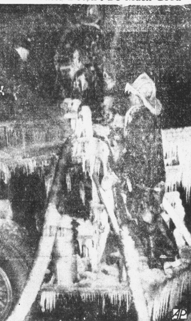
Water from these firemen's hoses literally are frozen assets. Frigid temperatures froze the water as quickly as it left the hoses, while a fire raged through a three-story wooden building housing a glass company. Damage was placed at $25,000.
