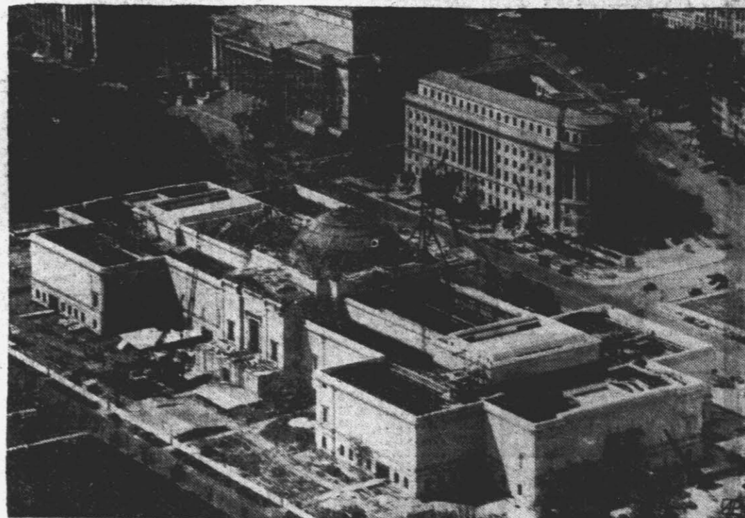
NATION'S NEW ART GALLERY —Here's a view of progress on the national art gallery in Washington, D. C. In rear are the apex, or trades, building and the archives building (left).
