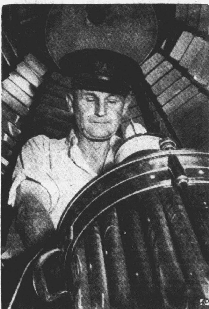
STILL BURNING KEROSENE —At the 85-year-old kerosene lamp of Point Conception light near Santa Barbara, Cal., one of the few remaining lighthouses not electrified, stands First Assistant Keeper Charles Hellwig. Point Conception sheds its faithful gleam over those waters often called "graveyard of the Pacific." In 1927 fog, seven U. S. destroyers piled up in 1927 fog.
