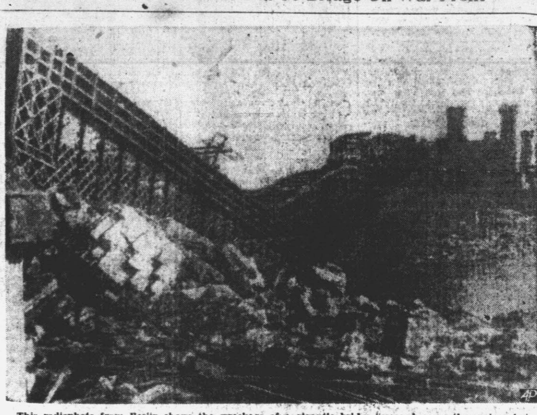
This radiophoto from Berlin shows the wreckage of a gigantic bridge "somewhere on the eastern battle front" after air bombers had finished with it. Because of censorship, no other details were available.
