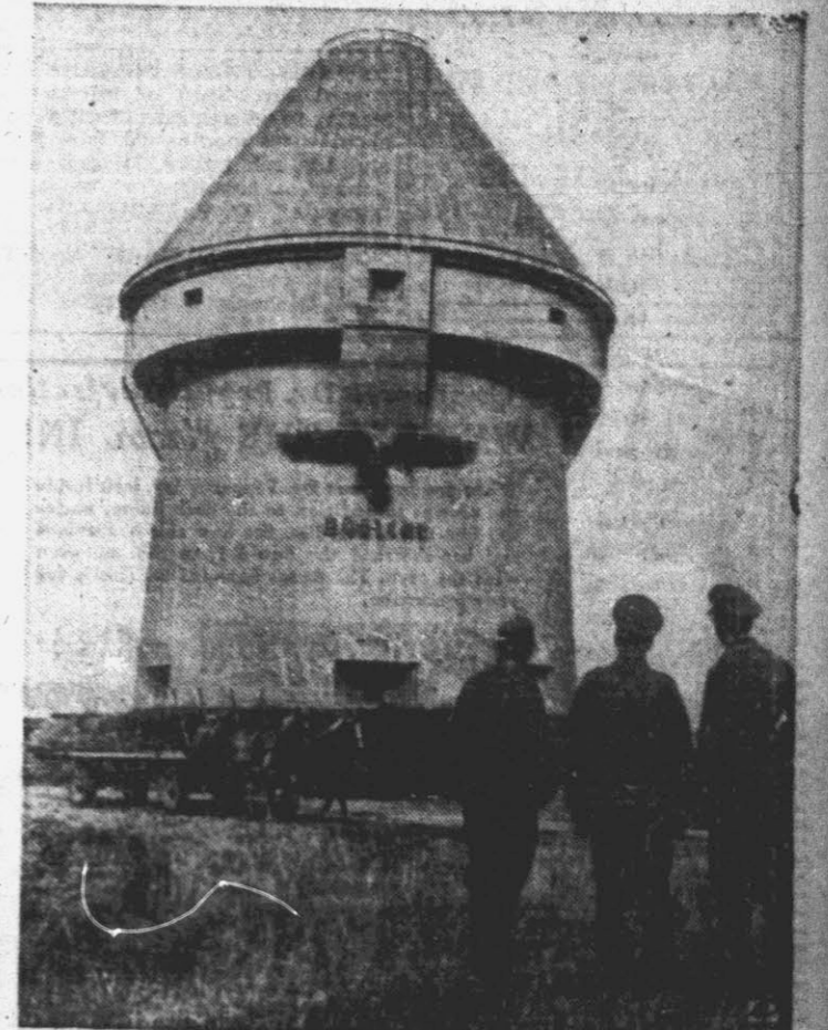
IT LOOKS LIKE A SILO —But appearances are deceiving. It's a tower of reinforced concrete along Germany's Siegfried line on her western frontier, designed to give shelter to 2,000 people. Nazi military spokesmen say it's "invincible." They contend it will withstand any attack from the sea.
