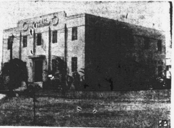
EARS FOR UNCLE SAM —Good reception is reported for above naval radio station NAU, recently rebuilt at San Juan, Puerto Rico, at a cost of $100,000. Naval strategists point out the value of NAU to the Caribbean defense plan.
