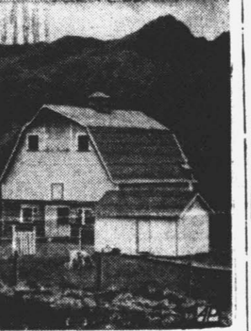
MODERN FARMS dot the valley now, though, with substantial buildings like the barn shown here.
