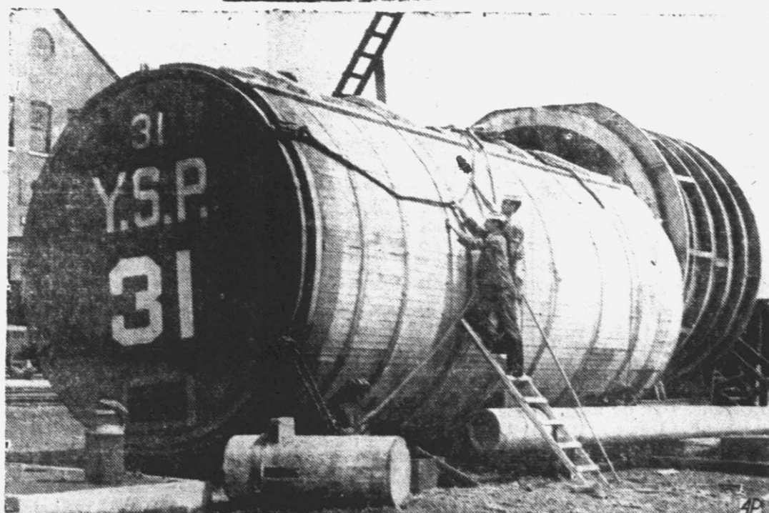
READY FOR LIFTING JOB —Workmen adjust one of the steel, oak-covered pontoons to be used in lifting the Squalus, the submarine which sank May 23 off Portsmouth, N. H.
