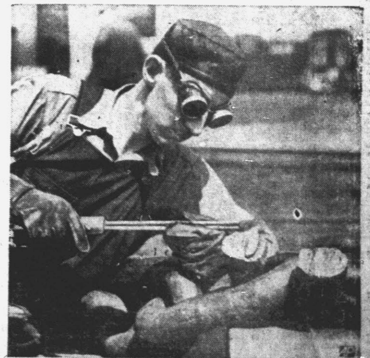
A LOOK AT LINKS —Five tons of chain with 2 1/2-inch-thick links (shown) will attach to pontoons in Squalus salvage.
