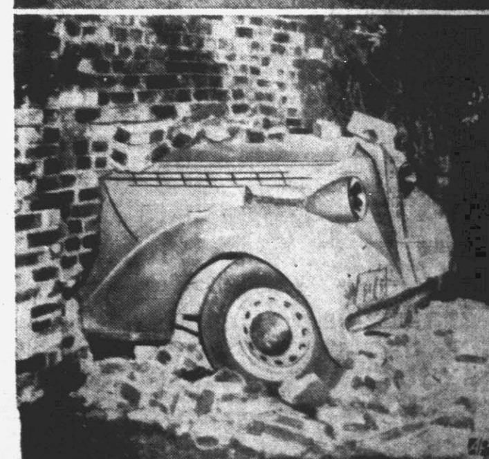
CAR... JAR... MARRIED! —The wall and the car suffered the most damage in this freak auto rampage at Sacramento, Cal., where the auto driven by Mrs. Maria Steiner nosed into this brick wall. Neither Mrs. Steiner nor the two persons with her were seriously hurt when the car, after a collision with another, bounced into a gas tank and then ran partly through wall.
