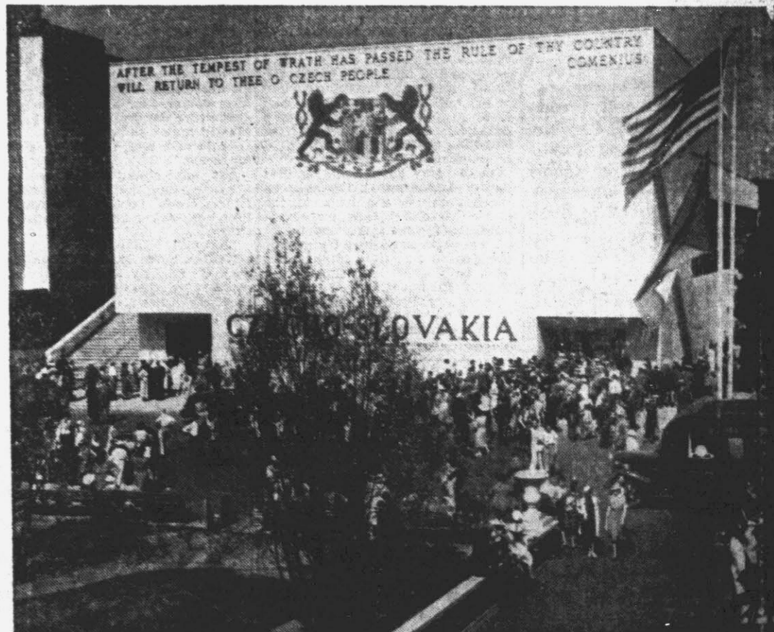
THE HOUSE OF HOPE —To thousands at the dedication of above Czechoslovakian pavilion at the world's fair, N. Y., this building symbolizes a dream that the country absorbed by Nazis will again find independence. A sign explains that the structure, though unfinished, is "maintained by its friends in America," and at the right a flag flies at half staff, mourning the country that lost its identity last March after aggression by Germany. Dr. Eduard Benes, exiled former president, and Czech Minister to U. S. Vladimir Hurban dedicated the building.
