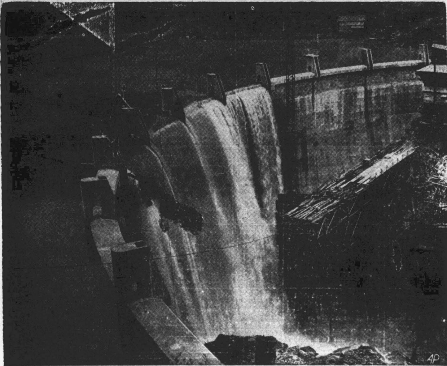
DAWN OF NEW DAY FOR HYDRAULIC MINING may bring a gold boom to land around Auburn, Cal., where this concrete barrier 155 feet high crosses the American river, as the first of a series of debris dams being built under the direction of army engineers. Before hydraulic mining was legislated out of existence in 1893 after years of strife between miners and farmers, it produced the bulk of the gold mined in California. The lake is intended as a settling basin for diggings unworked for years.
