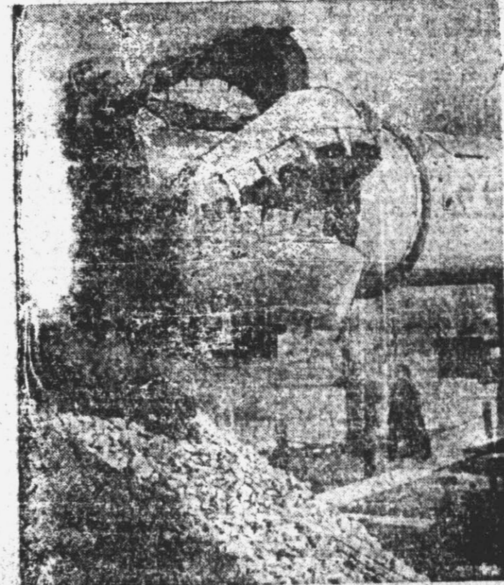
ANOTHER NAZI DRILL —this one, non military—appeared at the Leipzig fair. It's a "giant robot" which drills into sand and other material to be moved, like a giant borer. Attendees said that 70 tons of sand per hour could find its way through the tube, at right, and into a truck. Note the great teeth with which the drill bites into gravel or sand.
