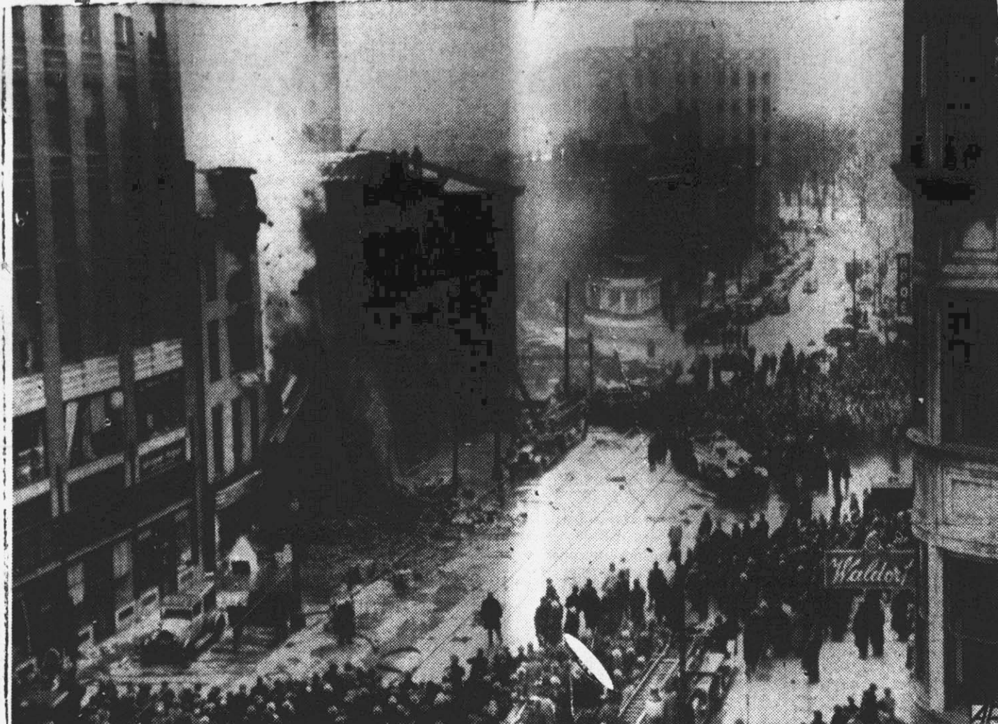
The collapsing wall of this Syracuse, N.Y., office building here piles additional tons of debris on top of the bodies of eight firemen who were plunged from the third story to the basement by the cave-in of the room. A ninth fireman, similarly trapped, was rescued. Although hope was abandoned for the eight men, rescue crews continued to search the smoking ruins.
