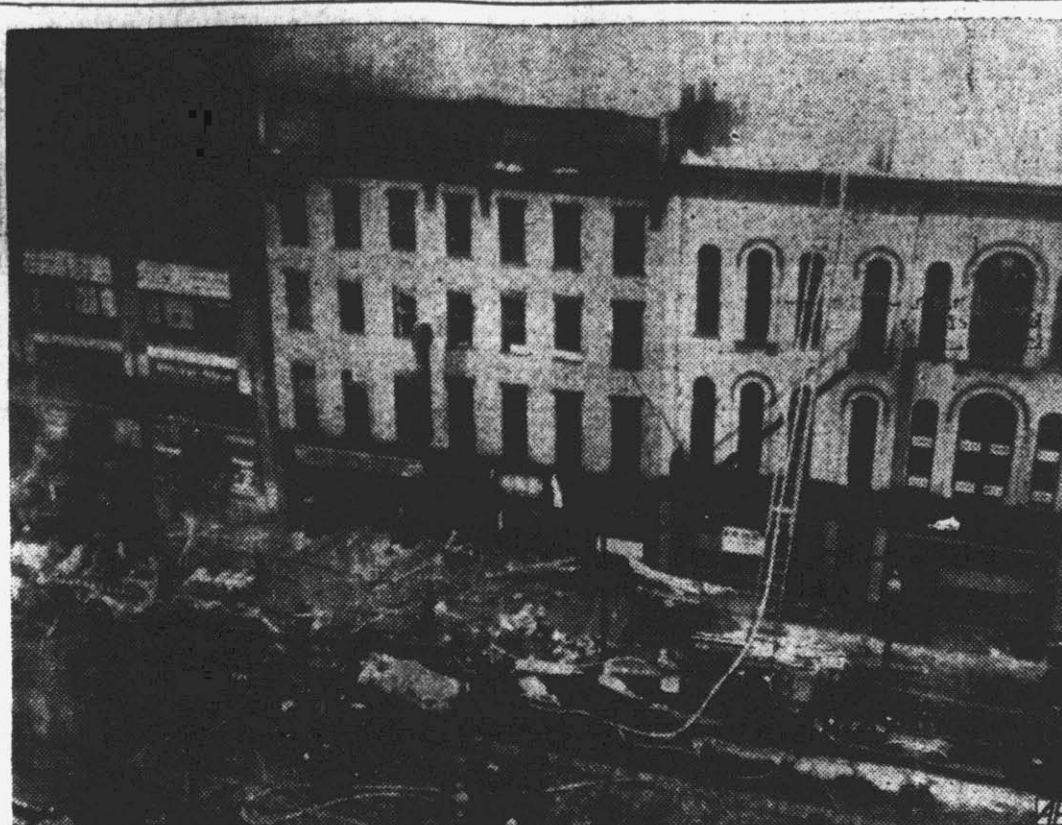
Collapse of the roof of this five-story Syracuse, N. Y., office building plunged nine firemen, who were fighting fire on the third floor, into the basement. An hour later rescue workers removed one, whose condition was critical. Efforts to dig out the other eight were hampered by danger of collapsing walls, which had to be braced.
