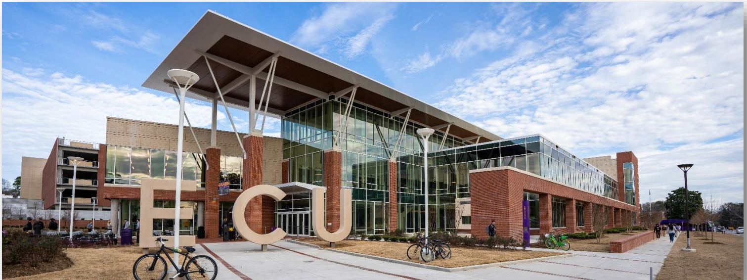
Main Campus Student Center 501 East 10 th Street, Greenville, NC
