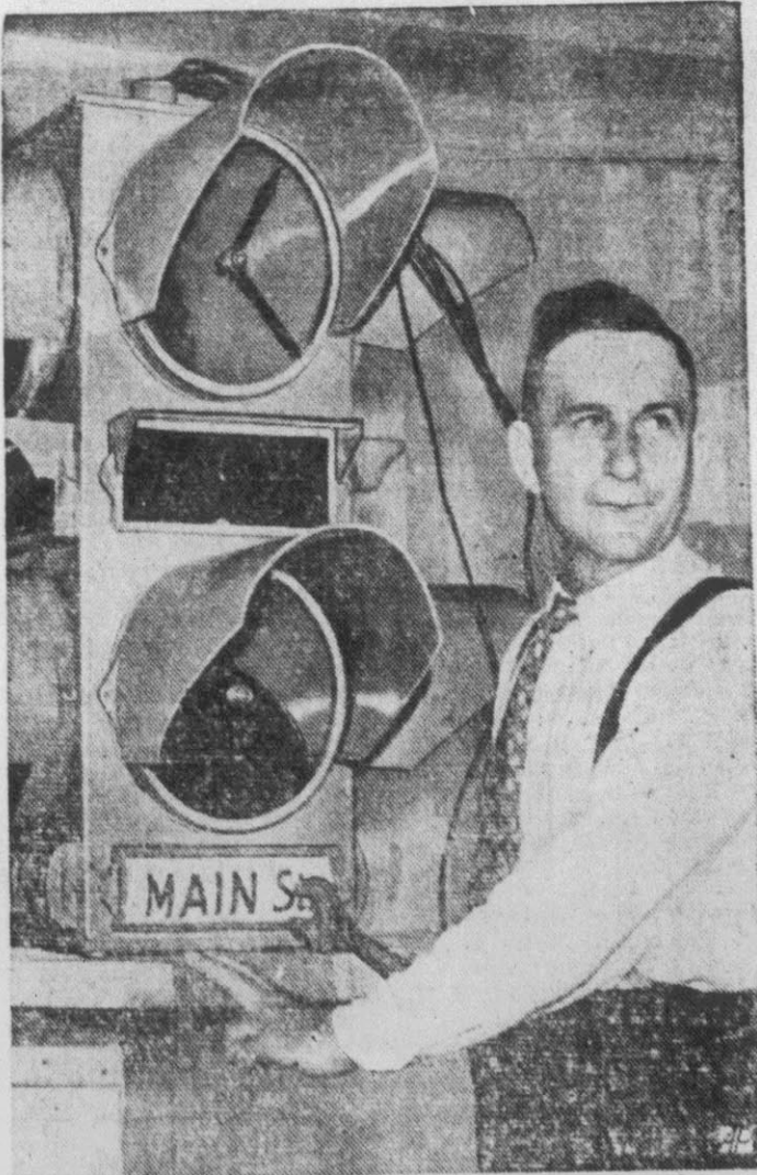
STOP CLOCK to keep pedestrians from being trapped by light change was invented by the Ebert brothers of Kenmore, N. Y. Clock hands in face of red signal tell when light will change.
