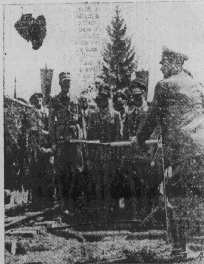
'EUROPE'S LARGEST' is Nazi claim for waterpower plant begun at Zell-on-lake by Goering, who turned first spadework.
