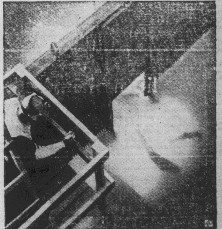
FISHY CENSUS is taken by counters as Columbia river salmon pass over white platform, using the $6,500,000 fishways to get upstream at Bonneville dam, a $52,000,000 government project. The fish climb about 63 feet, passing the dam.
