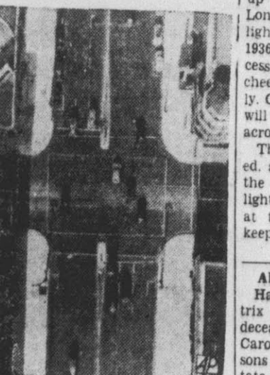
3. And here is picture made from the balloon at 300 feet. It shows an intersection with traffic lanes and safety islands.
