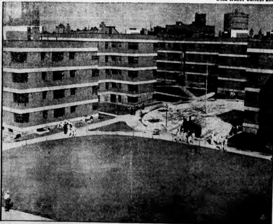
AND CHANGES LIVING HABITS for hundreds of former city slum dwellers. This is a portion of Williamsburg, largest slum-clearance project in the nation, built at a cost of $13,452,000 to replace 12 square blocks of over-crowded, worn-out tenements in New York City. Here eventually 1,600 families will live in apartments with all rooms outside and every modern convenience in place of heatless, often windowless, squalid rooms.
