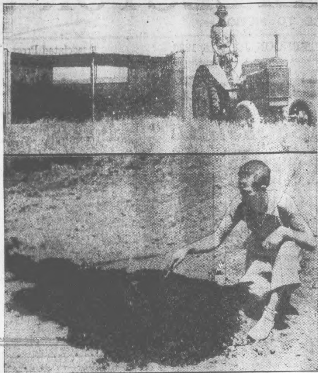
Partial relief from grasshoppers swarming over the drought-stricken middlewestern states is being furnished by this tractor-drawn trap (top) which is killing millions of the pests in the Fairfax district near Kansas City, Mo. As the trap moves over the fields, hoppers fly into it and are caught in an oil bath. Below, Bill Patch examines a pile of grasshoppers caught by the trap. (Associated Press Photos)
