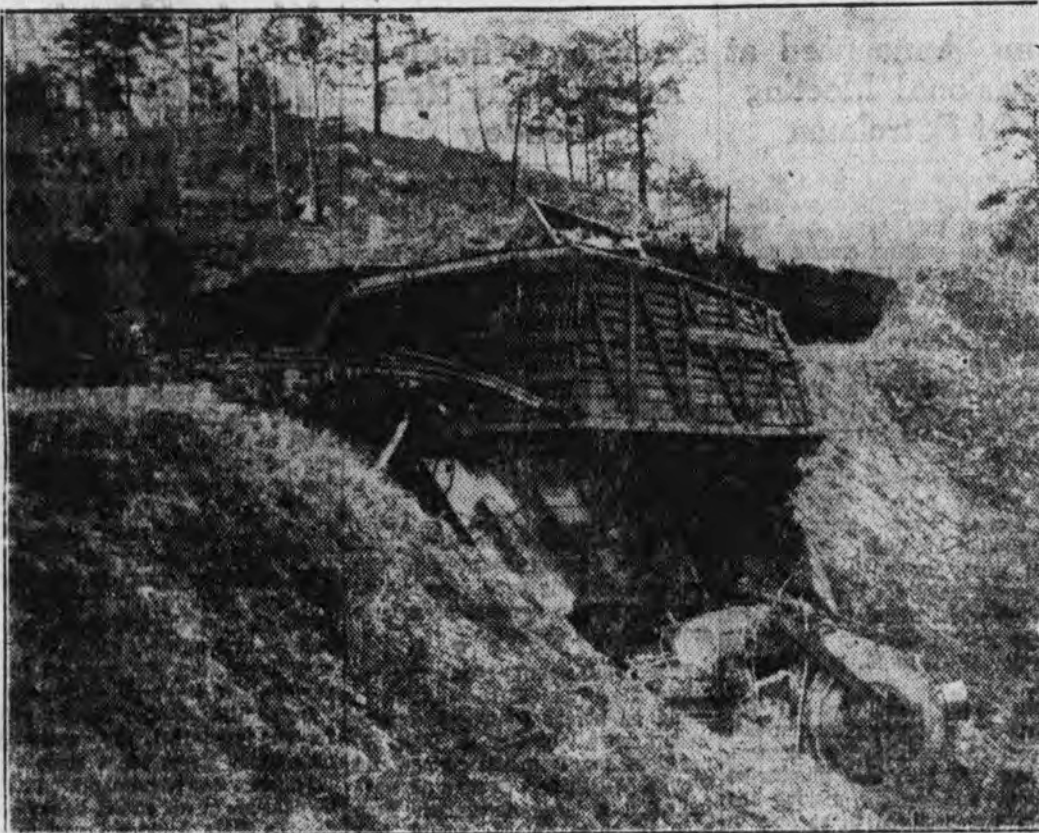
Two trainmen, brakeman J. H. Brown and Fireman Frank Kenamer, were killed near May-lane, Ala., in the wreck of a freight train caused by flood water. The locomotive, which can be seen buried in the ravine, and a number of cars plunged from the track undermined by the torrents. (Associated Press Photo)
