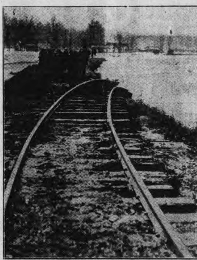
Torrential rains in east central Mississippi flooded streams, temporarily paralyzed railroad traffic at Meridian and marooned Yazoo and Mississippi Valley passenger train No. 210 about 40 miles west of the city. This picture, showing a section of the G. M. & N. railroad washed away, illustrates why trains didn't operate. (Associated Press Photo)
