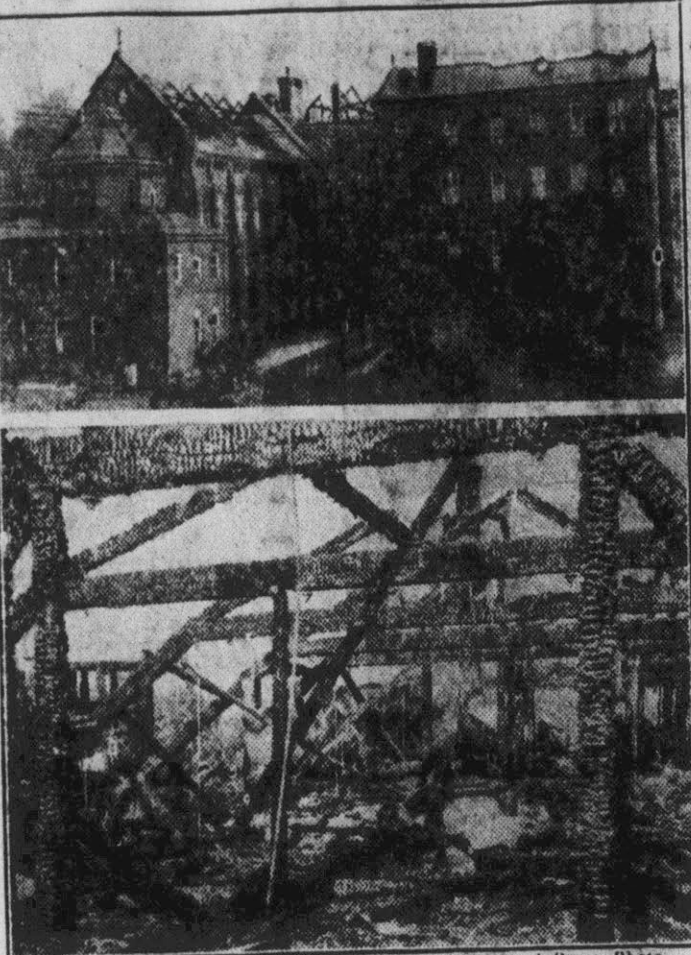
Associated Press Photo The Little Sisters of the Poor Home for the Aged in Pittsburgh, Pa., after it had been swept by a fire which resulted in 40 deaths. More than 200 were injured. Lower picture shows the ruins of the third floor where many of the inmates perished.
