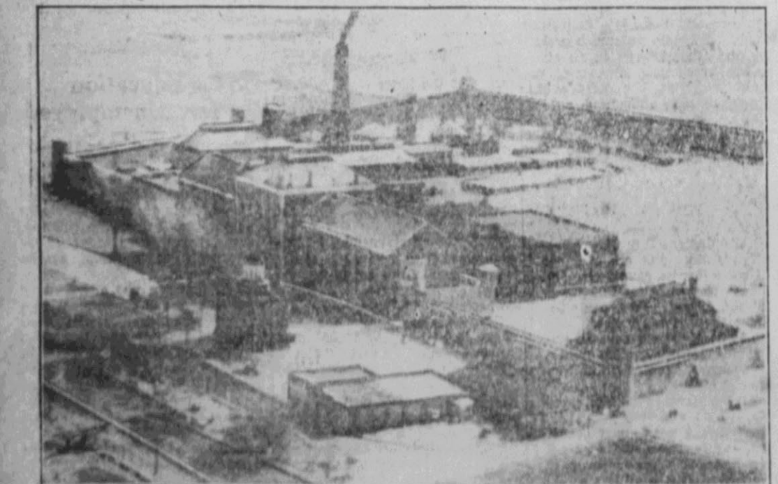
Above is an air view of the New Mexico state penitentiary at Santa Fe where Albert B. Fall, former secretary of interior, will serve his sentence of a year and a day for bribery. The cell blocks flank the central administrative unit, shown at the entrance to the prison. The building behind the right cell block is the prison hospital.
