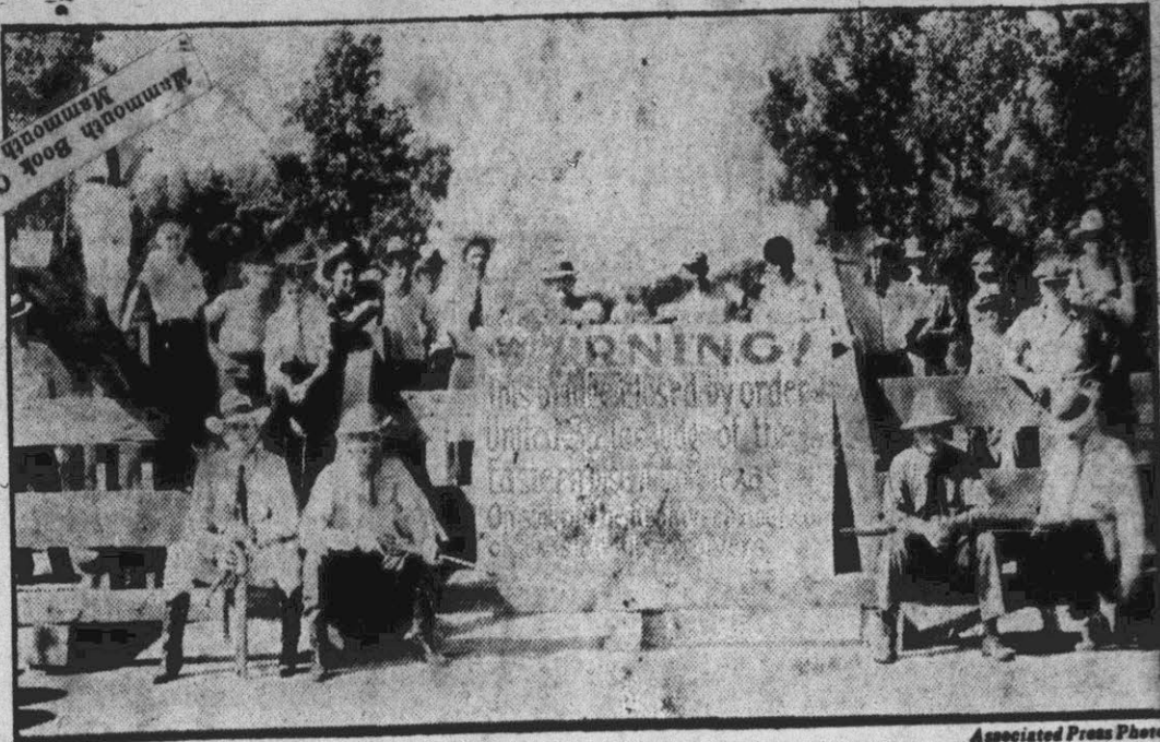
The new free bridge over the Red river between Denison, Tex., and Durant, Okla., became the center of a dispute when Gov. W. H. Murray of Oklahoma objected to the fact that Texas had not opened the bridge. After Murray ordered the bridge barrier torn down, Gov. Ross Sterling of Texas ordered Rangers to the scene. They are shown guarding the rebuilt barrier at the Texas end of the bridge.
