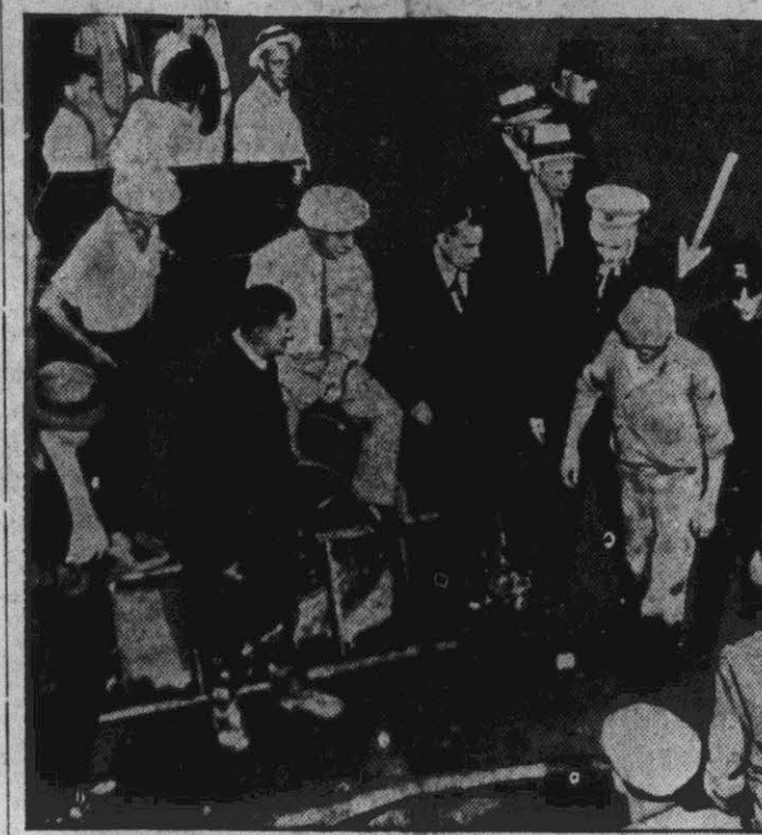
The first of 11 workmen trapped 37 feet underground when heavy rain flooded a section of heating tunnel in Milwaukee is shown being rescued by firemen after six hours imprisonment. All were saved.
