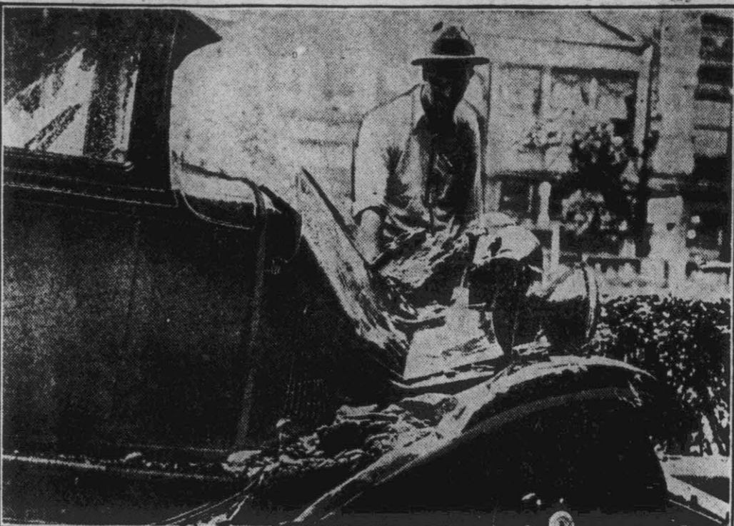
The late June heat wave was broken with a vengeance at Louisville, Ky., when a rainstorm, accompanied by a strong wind struck the city. Picture shows damage done to an automobile when a rock was hurled from the cornice of the Jefferson county courthouse.
