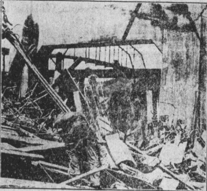
Two men were hurled to death near Carthage, Tenn., when a 40-foot span of a concrete bridge under construction collapsed. Five other workers were injured in falling with the wreckage.
