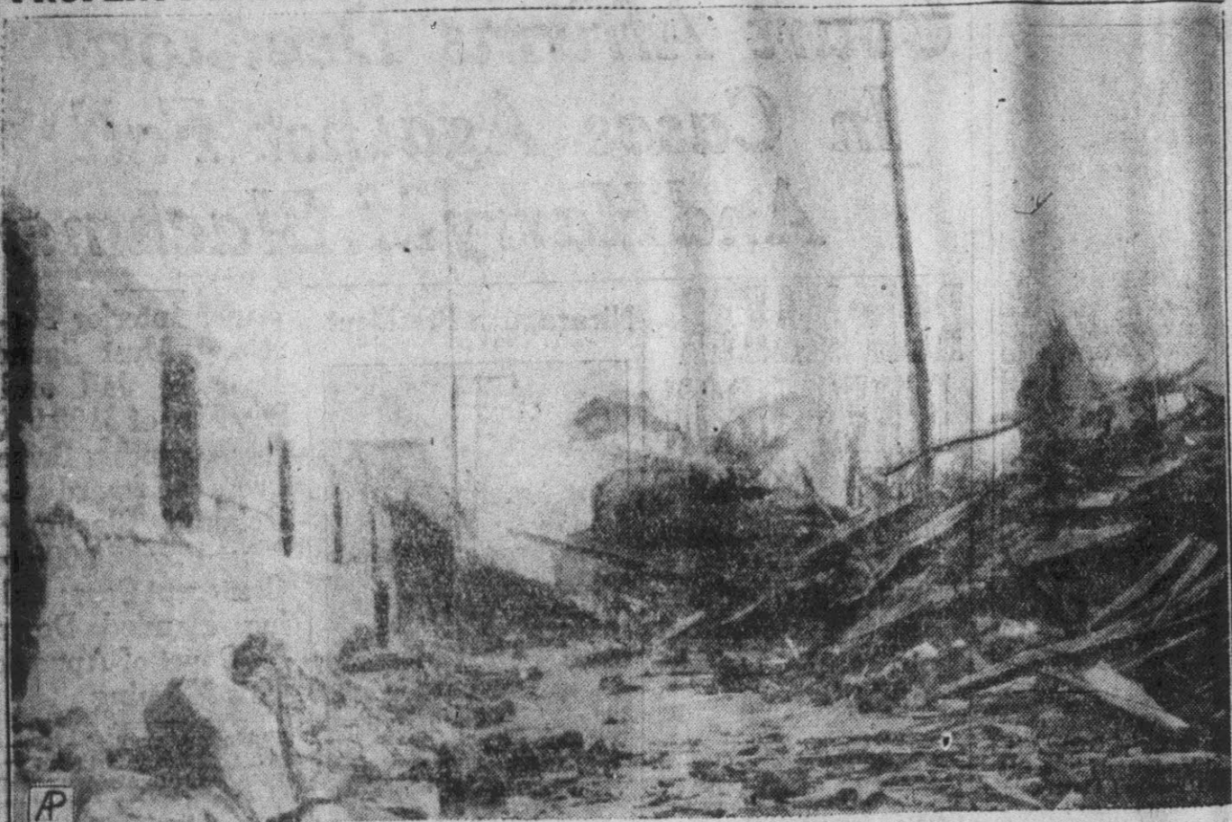
This Associated Press photo shows one of the principal streets of Managua, Nicaragua, practically destroyed by an earthquake, which caused the loss of 2,000 to 5,000 lives and property damage of more than $70,000,000. American refugees, including 150 women and children, were being removed from Managua by airplane, while American surgeons had set up improvised operating rooms wherever they could find a building to house them.
