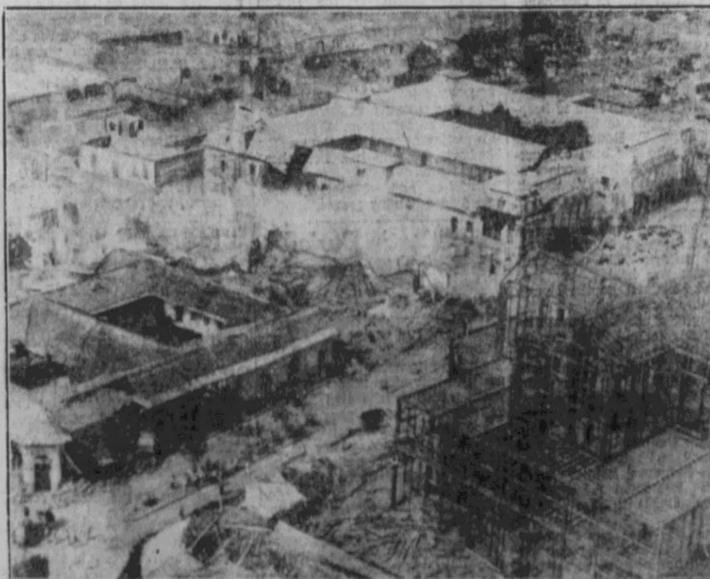
Associated Press Photo The smoking ruins of Managua, Nicaragua, are shown in this air view of the city taken while flames consumed wreckage left by terrific earthquake shocks. How buildings were leveled by the quake and walls shattered is shown by the photo. The death toll is expected to reach 2,000 while property damage was so heavy it is doubted if the city will be rebuilt.
