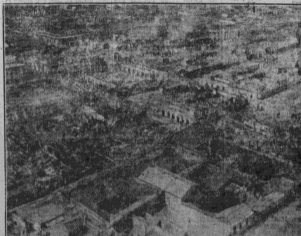
Associated Press Photo This air view of Managua, Nicaragua, taken after the earthquake that damaged or destroyed virtually every building in the city, shows a section of the business district in ruins. First estimates placed the property damage at $70,000,000.
