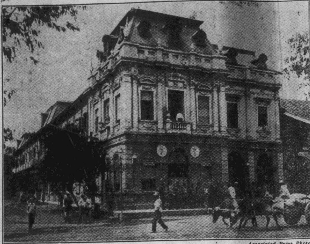
Here is the National theater in Managua, the capital of Nicaragua, which was devastated by an earthquake. The quake, and a fire which followed, caused a heavy loss in the capital and took a death toll at first estimated at half a hundred.
