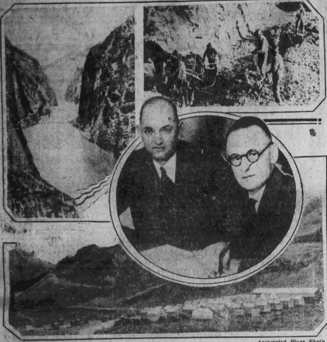
Actual work has started on the $165,000,000 Hoover dam project, which, when completed, will be the largest in the world. Upper left: The dam site in Black canyon, Colorado river, in the Nevada wastelands. Upper right: Workmen excavating for the power house which will furnish electricity for construction work on the dam. Frank Crowe (left) and Walker Young, construction engineer, U. S. bureau of reclamation, are in actual charge of construction. Below is the tent city erected by workmen near the dam site.
