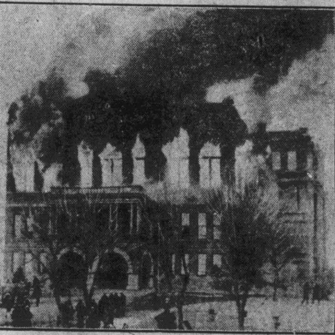
Flames devouring the North Dakota capitol building at Bismarck. Practically all of the official records and historical documents were destroyed. The building was erected in 1894 when the Dakotas were territories.
