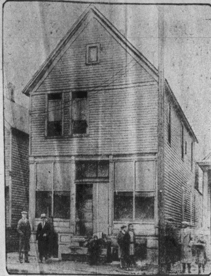
Rooming house at Whiting, Ind., where 7 men celebrating Christmas were burned to death as fire gutted the building at dawn. One man saved his life by leaping from second story window, left.
