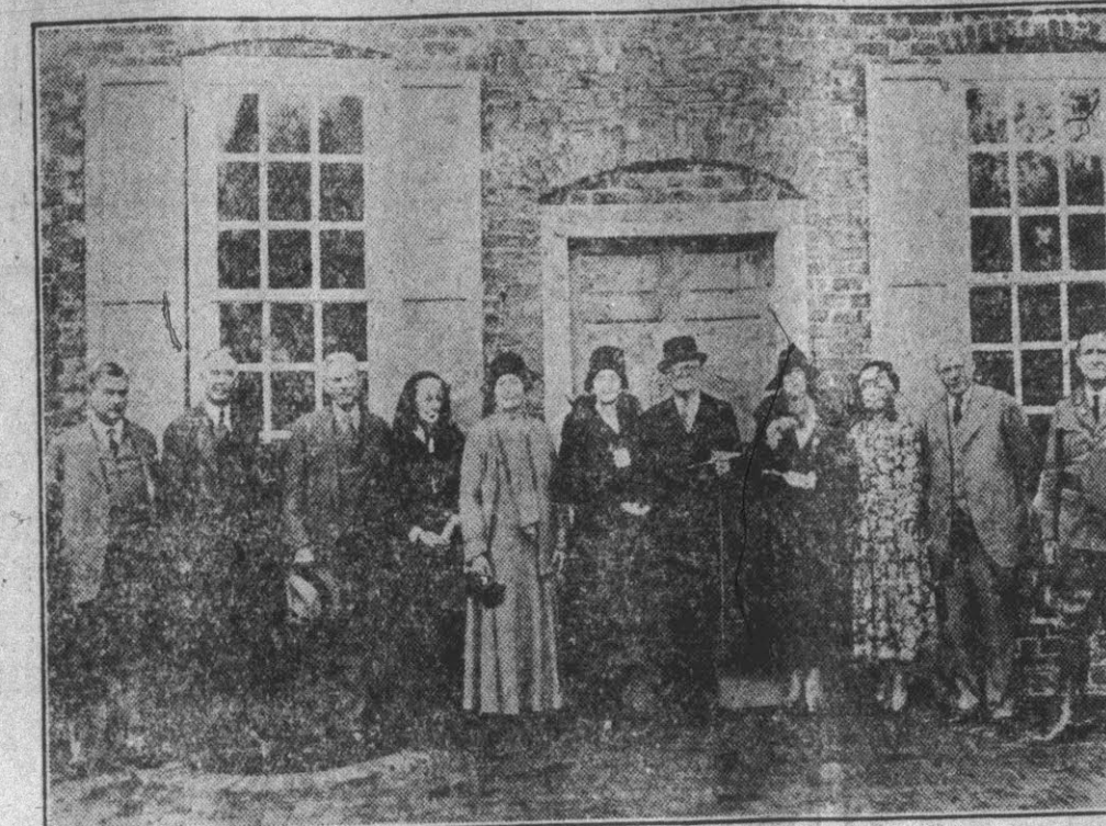
The old custom's house at Yorktown, Va., built in 1706, has been made a national shrine, after its restoration by Mrs. Arthur Kelley Evans, of Atlanta, and Hot Springs, Va. Governor John G. Pollard, of Virginia (center, wearing derby) made the dedicatory address at the ceremony.
