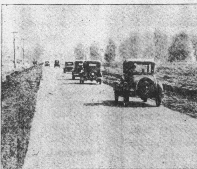
Associated Press Photo This is an experimental section of iron highway in Sangamon county, near Springfield, Ill. Bricks are laid on metal sheets.
