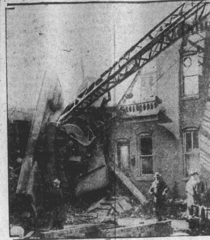
This large steel crane, topping off an elevated railroad track, fell 20 feet and crushed a Detroit flat building.
