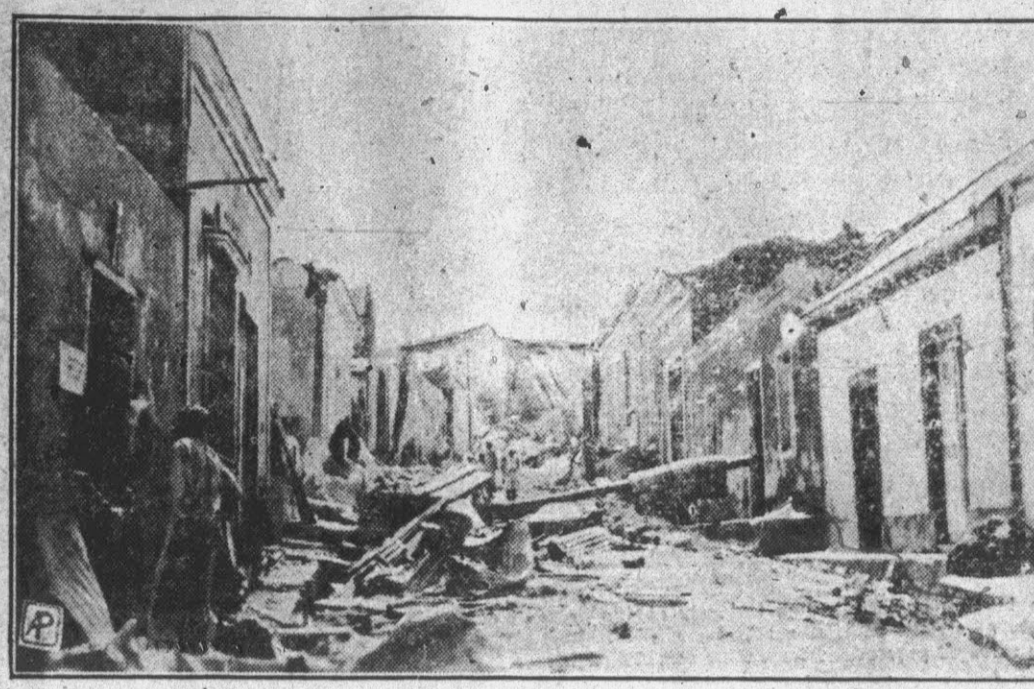
Associated Press Photo Observers estimated that 90 per cent of all buildings in Santo Domingo were wrecked by the tropical hurricane which struck the city, taking 4,000 lives. This picture shows one of the principal streets choked with debris.
