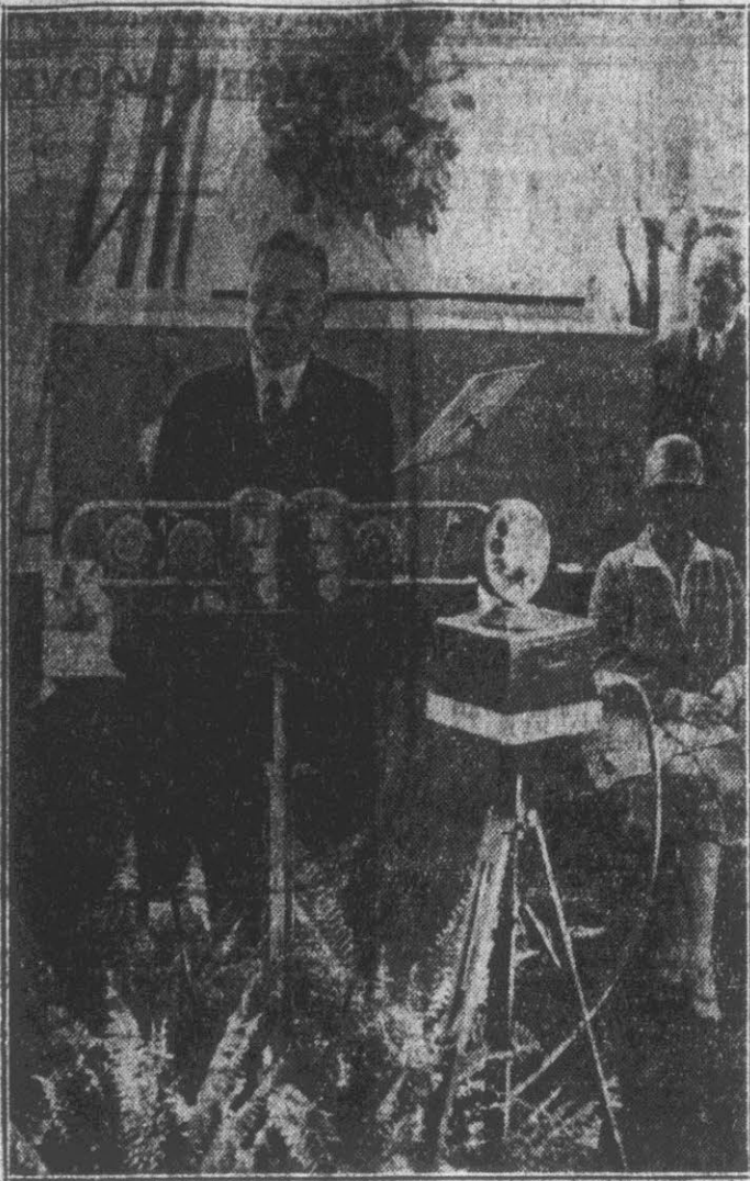
Laying the cornerstone of the new department of commerce building, President Hoover made a brief address. Mrs. Hoover is on the right. The cornerstone is in the background.
