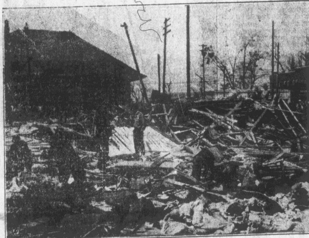
Duncan, Miss., was recently visited by a storm. Streets were littered with debris from which 17 bodies were removed. A railroad station is at the left.
