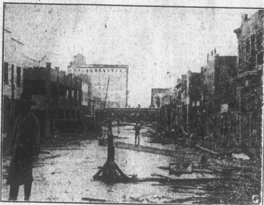
West Palm Beach's principal street, Clematis avenue, showing damaged buildings before workers began clearing debris left by the hurricane.
