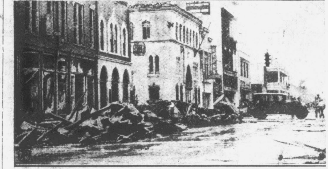
Property was destroyed and lives endangered by falling walls and wind-blown debris during the height of the Florida storm at West Palm Beach. The photo shows the wreckage of an automobile caught beneath the tumbling brick of a building adjoining the Western Union office.
