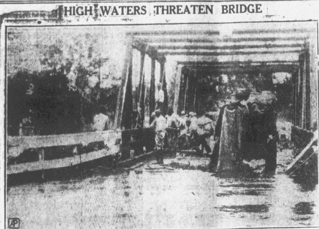
A road gang in Florida is shown here endeavoring to save a bridge menaced by flood waters. Reinforced abutments and cables from bridge to shore saved the structure from being swept from foundation.
