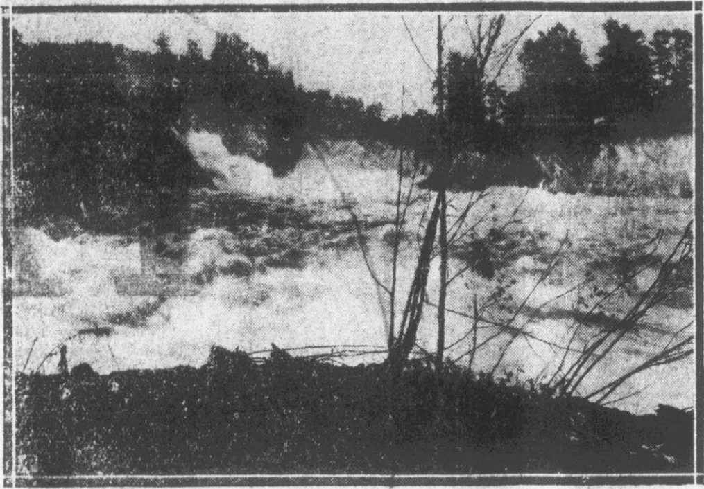
Where recent storms and rains near Bridgewater, N. C., caused the waters of Lake James to rise to a point which menaced the safety of surrounding country, the flood gates which dam the outlet were opened to relieve the danger.
