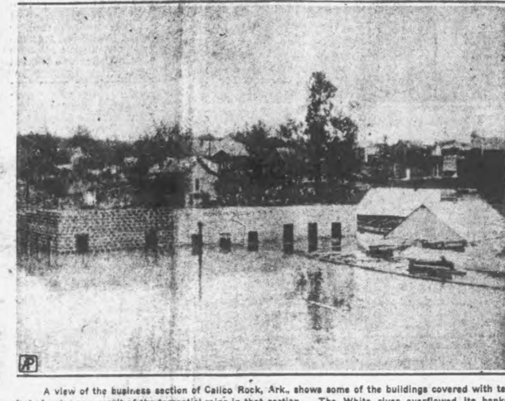
A view of the business section of Calico Rock, Ark., shows some of the buildings covered with feet of water as a result of the torrential rains in that section. The White river overflowed its banks, covering several sections of the town from a depth of two to ten feet.
