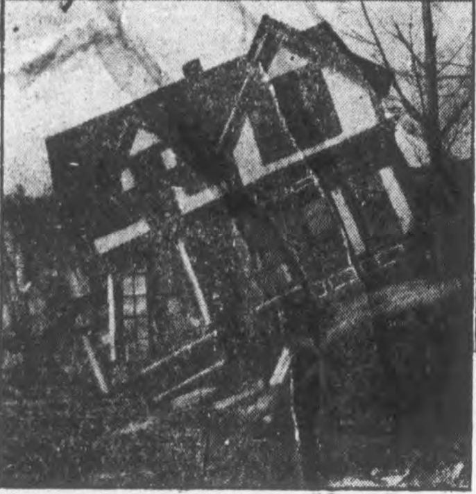
The sturdy construction of New England homes was shown when many houses, swept for rods or miles by flood waters, landed almost intact. The home below at Bethel, Vt., was tipped on edge but did not crack up. The Mays home (above) at Bolton, Vt., was carried three-fourths of a mile and set down in a railroad track without even losing a bundle of shingles perched on its slanting roof.
