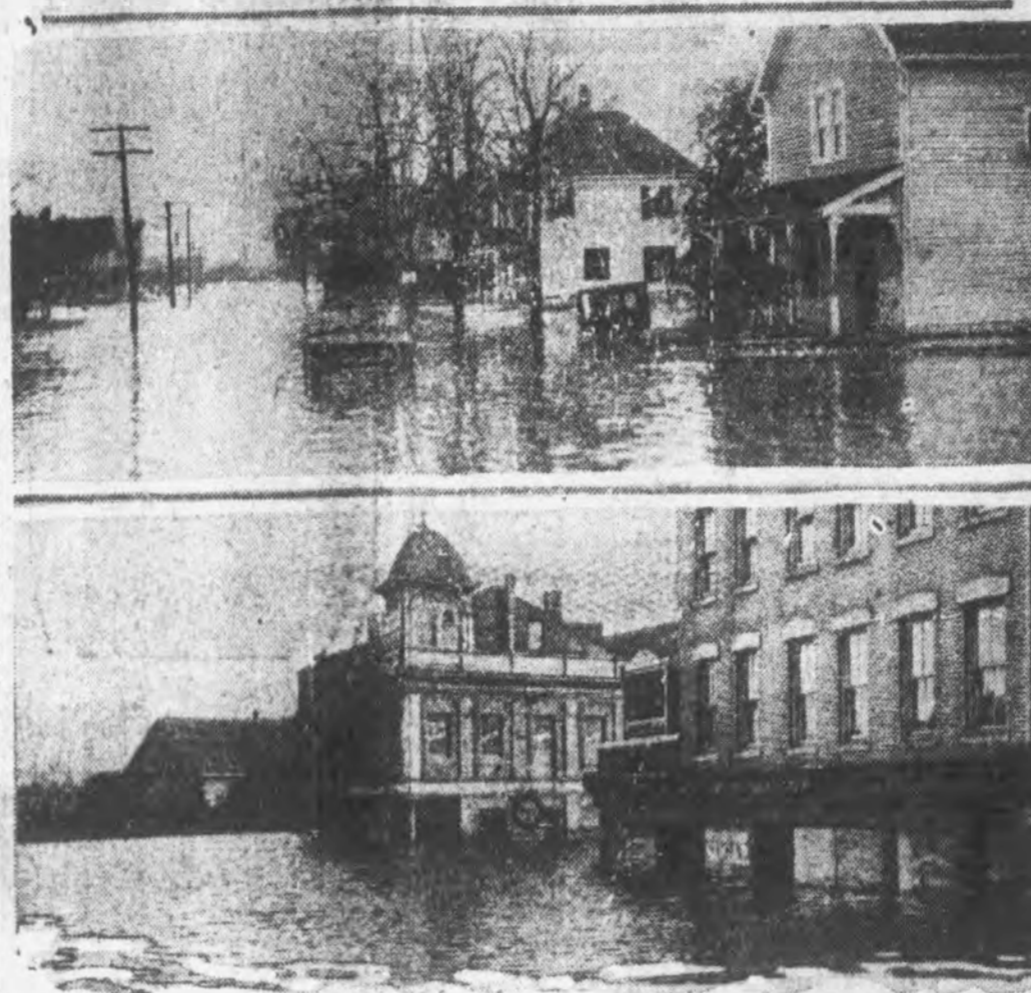
Two views of submerged portions of East Hartford, Conn., after being inundated by torrents that ravaged New England: Top—Depth of water may be realized by noting that top of an auto barely shows above "lake." Bottom—View of State street, business center, showing how high water has risen against buildings.
