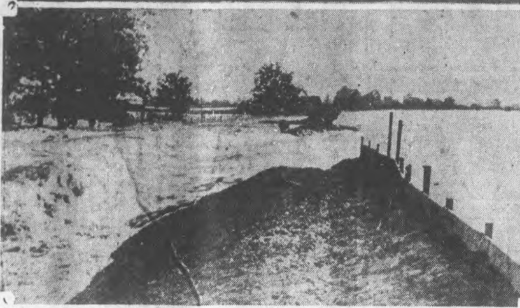
The Mississippi River is cutting a new channel to the sea through the Louisiana "sugar bowl." Picture shows one of the many breaks in the levee through which water, estimated at 600,000 cubic feet a second, is pouring.
