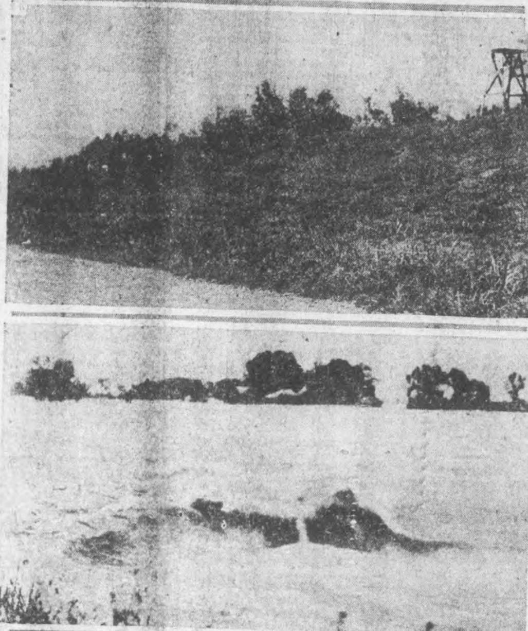
New Orleans appears to be safe now from flood waters of the Mississippi. The levee at Poydras, Miss., was dynamited, permitting water to flow over the St. Bernard marshes to the sea. Top picture shows the spot on the levee where half a dozen small blasts of dynamite were exploded to tear a small hole through. The force of the flood is eating a wide gash in the embankment, and the lower picture shows the break as it is today.
