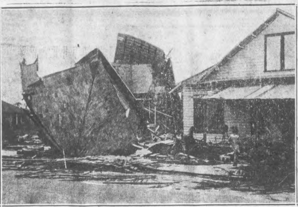
House were turned upside down by the force of the hurricane that spread death and destruction through Florida. This shows some of the damage at Miami. (Copy right 1926, International Newsreel).
