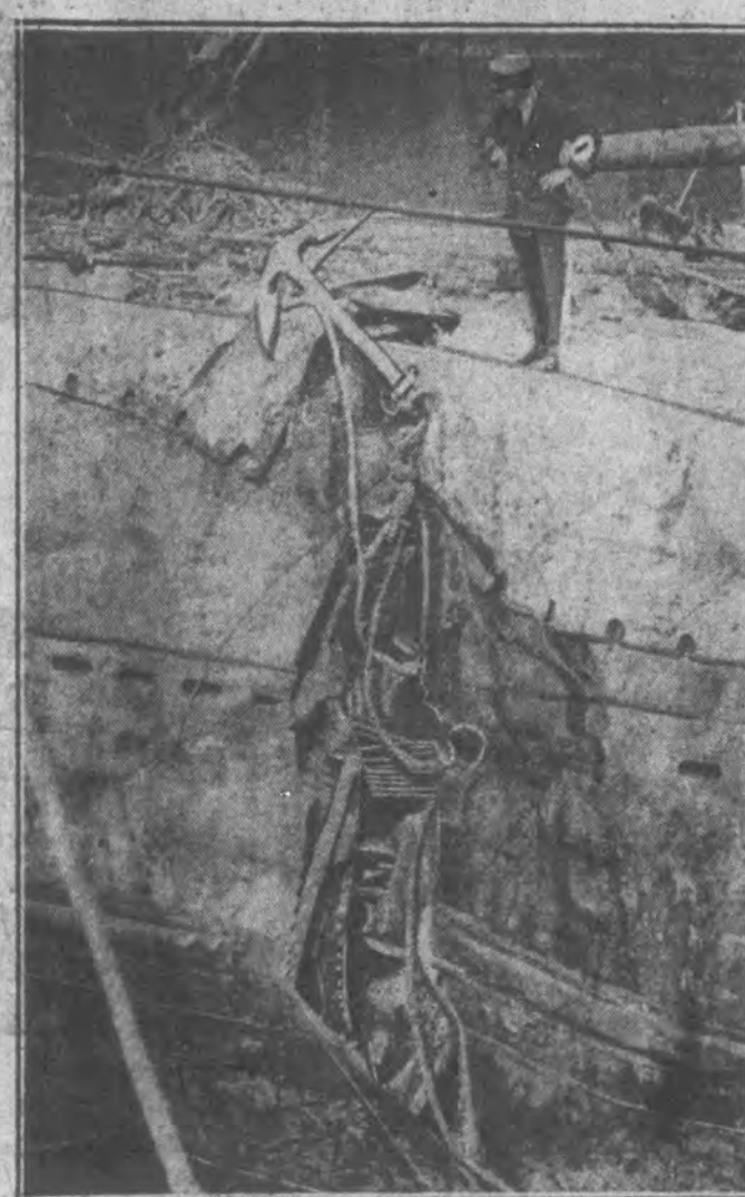
Here is the hole that the City of Rome tore in the S-51, sending the submarine to the bottom. The picture was taken at the Brooklyn Navy Yard, where the sub was in drydock.
