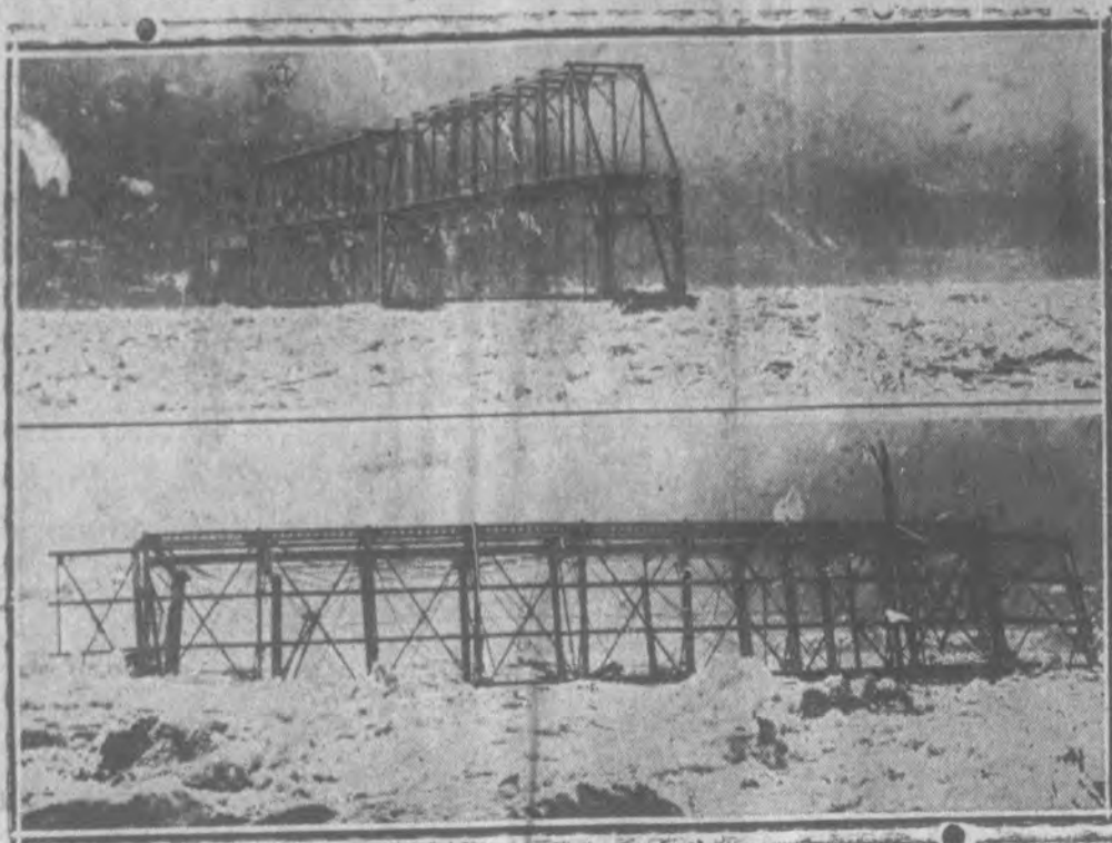
These two views show how the Allegheny River ice jam crushed the Big Rock Bridge, near Franklin, Pa. Above is shown the half of the bridge which withstood the tremendous pressure. Below is the other half which was swept downstream with the great masses of ice.
