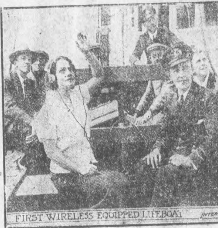
Photo shows Donita Castlegrand as she signals to the bridge of the S. S. Orbita to lower away—and the Orbita's radio-equipped lifeboat takes to the water. This lifeboat is the first of its kind and is a new departure in safety first at sea. There is a specially trained crew to operate the portable radio which, in case of accident to the steamer, would at all times be able to maintain communication with rescue ships.
