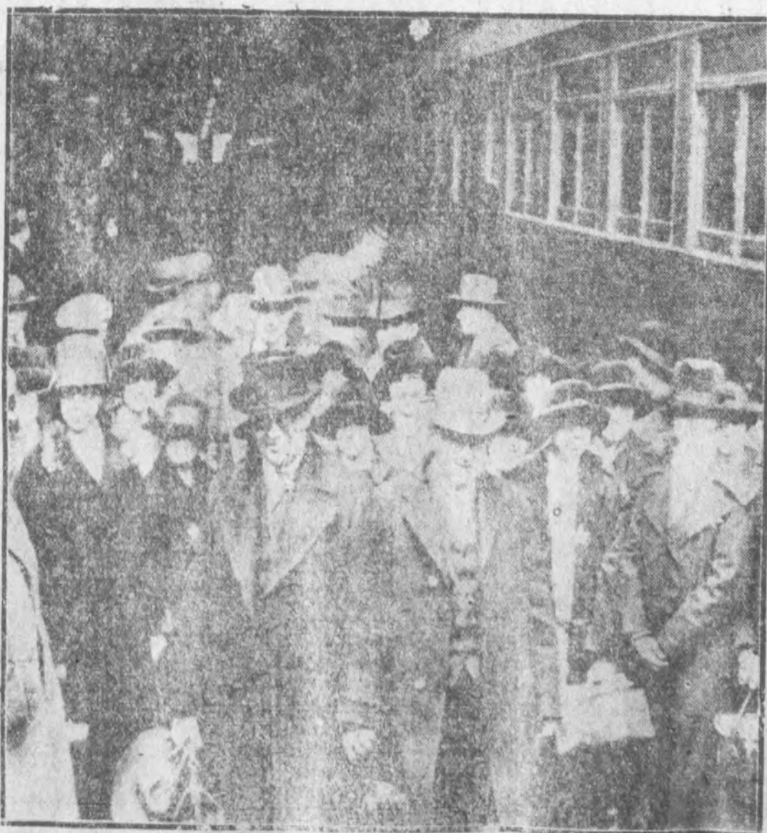
Relief doctors and nurses leaving Chicago for tornado devastated section of Illinois. Photograph transmitted from Chicago to New York by wire by American Telephone & Telegraph Co., copyrighted and supplied by International Newsreel.
